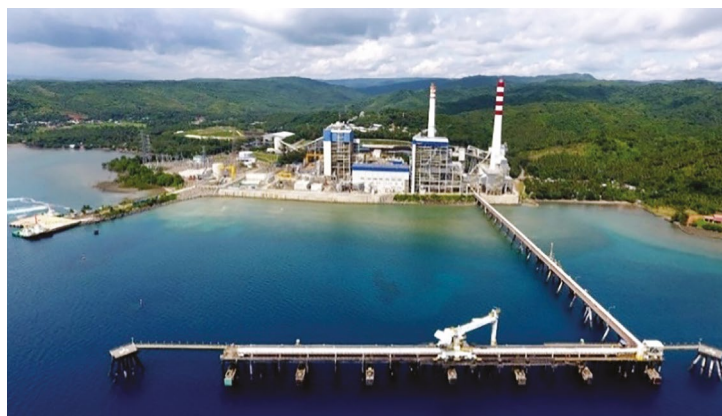
The 500-MW supercritical coal-fired power plant of San Buenaventura Power Ltd. Co. in Mauban, Quezon (source: tribune.net.ph)
