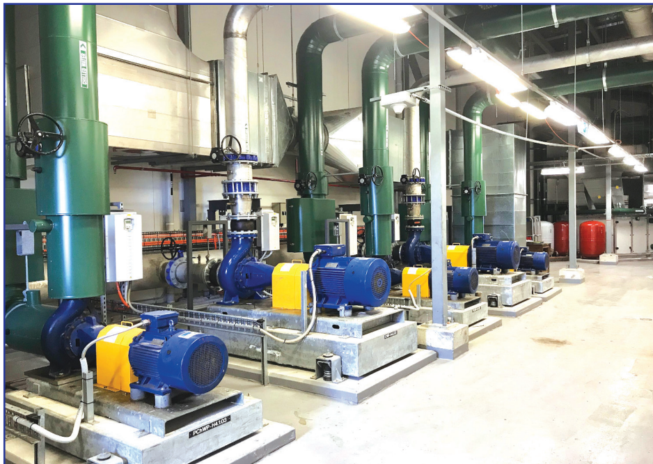
Photo shows chilled water pumps to circulate the chilled water.
