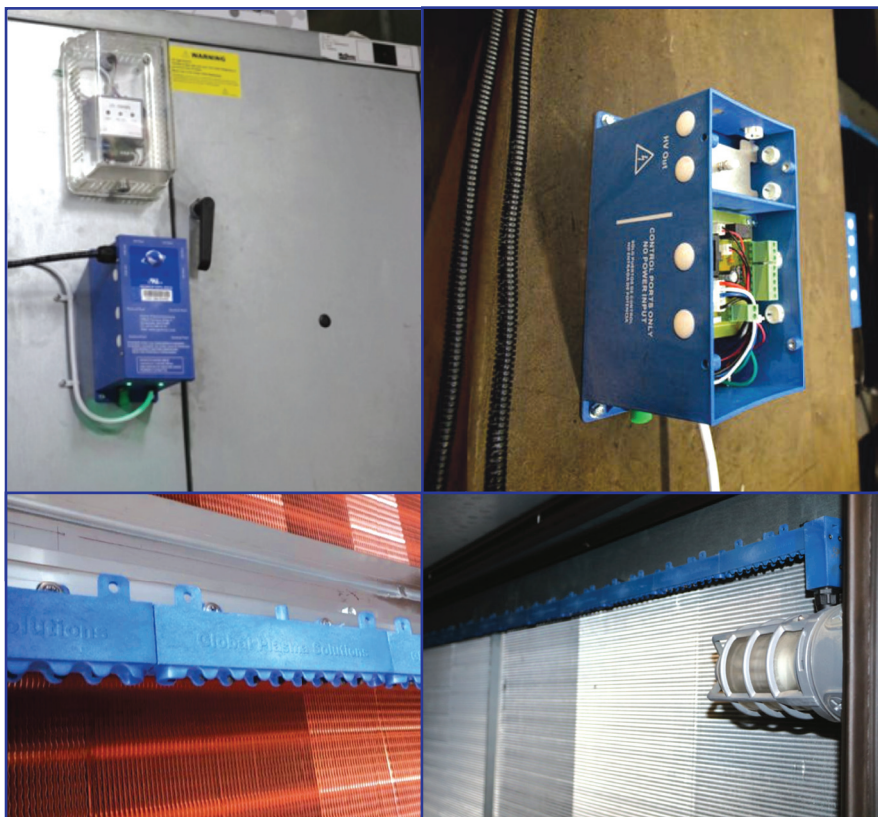
Acrylic Bi-Polar Ionization Tubes (replaced every 2 years)
