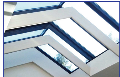
Skylight – roof opening covered with translucent or transparent glass or plastic designed to admit daylight.
