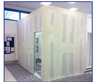
Demising Wall – an interior wall of partition used to subdivide one space from one another or from the common spaces.
