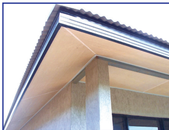
Soffit – connecting the top of an exterior wall to a projecting eave.
