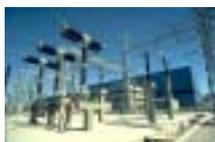
At the end of the high-voltage transmission line in town or city, bulk power or delivery point substation is connected. The power transformer in this substation lowers the voltage to subtransmission level.
