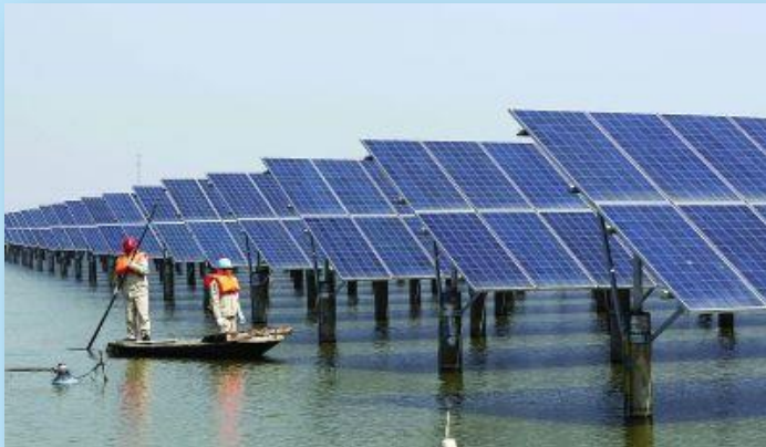
PV and fisheries integrated design
